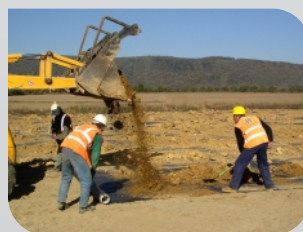
Belotín - motorway D47
