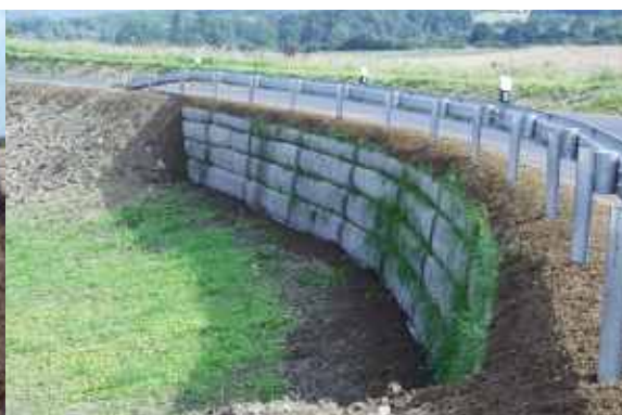
Placing of geogrids. Temporary formwork at the back
