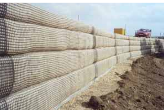
Final appearance of the reinforced earth structure
