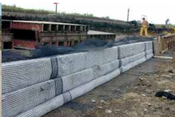
Placing of geogrids. Temporary formwork at the back
