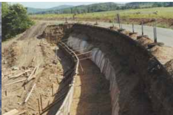
Excavated soil of the landslide with temporary formwork
