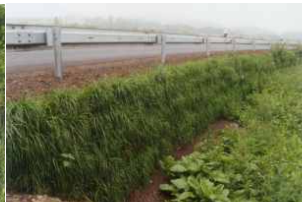
Reinforced earth structure with green facing (2000)
