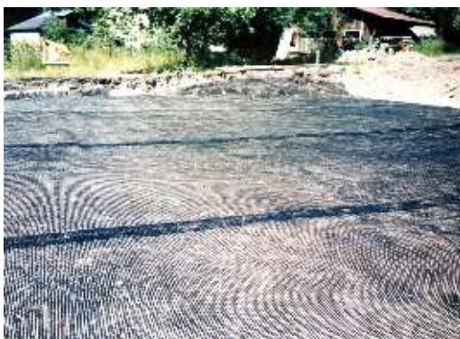
Armatex® G 55/30 geogrid laid on levelled and compacted layer.
