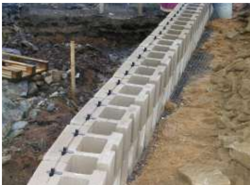
Plastic pins for fitting to adapted pieces, they also serve for anchoring geogrids.
