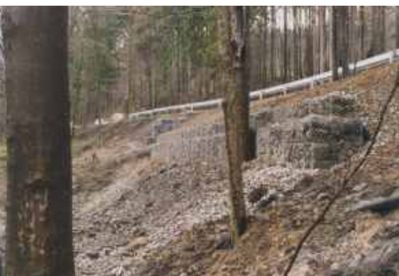
Fig. 4 Slope after maintenance
