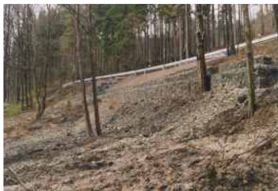
Fig. 5 Slope after maintenance
