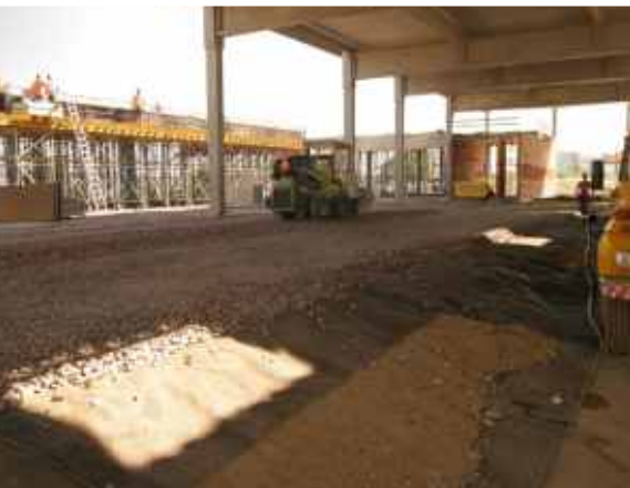
partial phase of construction
