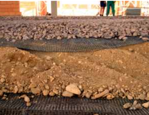
composition of construction strata
